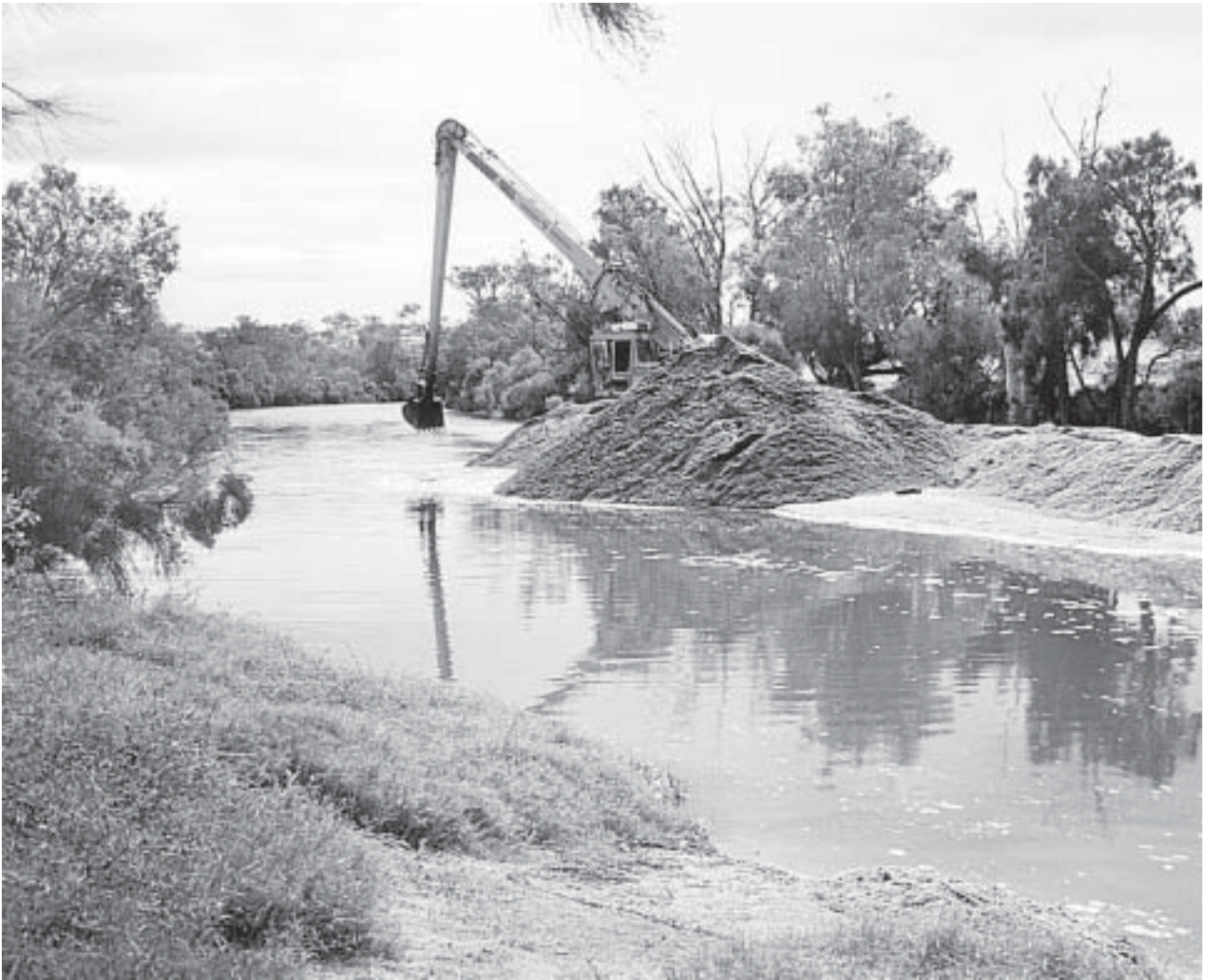
Photo 9. Excavation of sediments from the pool.
