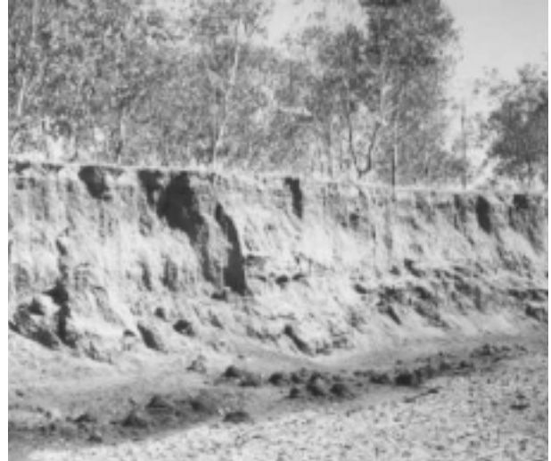
An example of severe bank erosion along Spencers Brook
