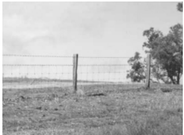
Fence condition: GOOD
