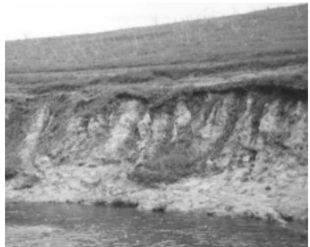
Bank erosion along Talbot Brook
