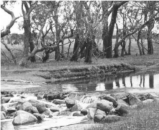
A man-made riffle provides a crossing point for stock and vehicles, acts as a sediment trap and aerates the water
