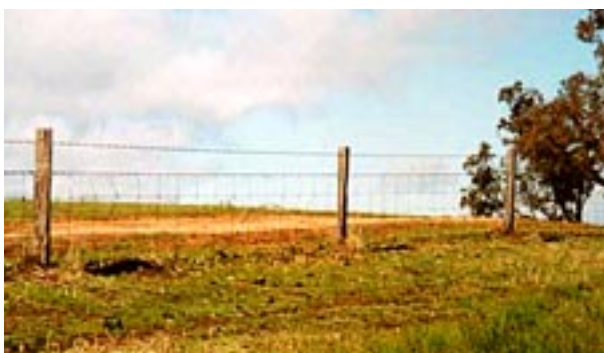
Fence condition: GOOD.
