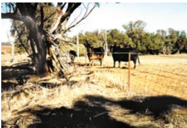
Fence condition: MODERATE.
