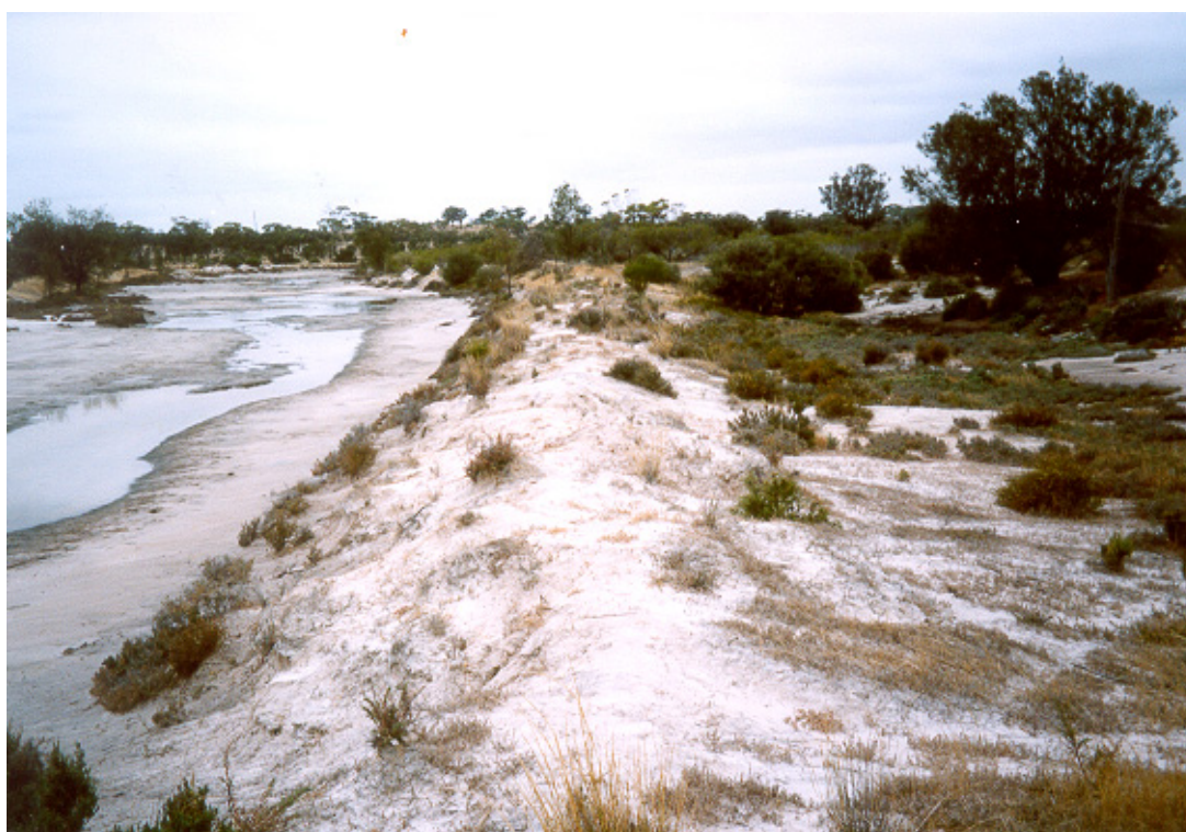
Levee banks were the most common form of earthworks within the riparian zone
