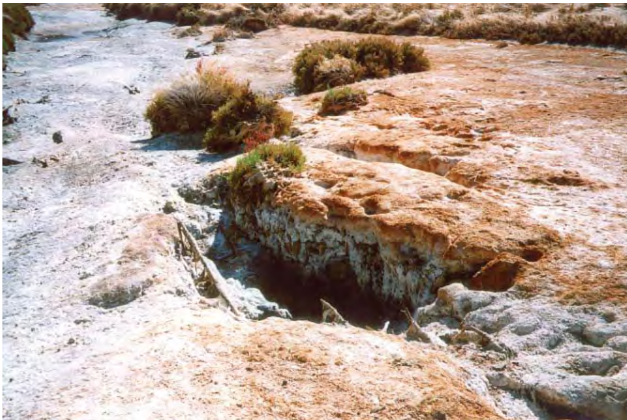
Photo: Consolidated silt within river channel
