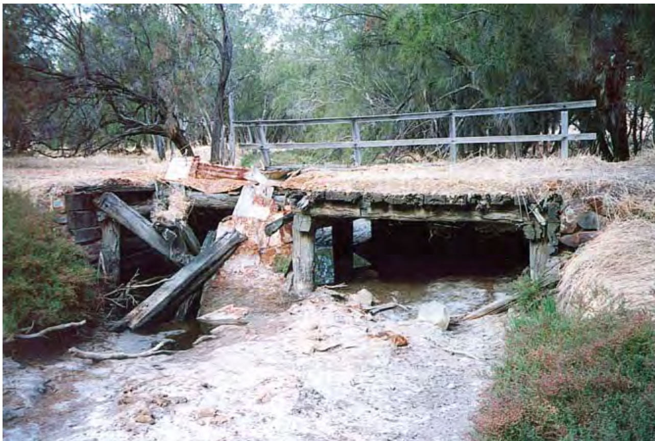
Photo: Crees Road Bridge (decommissioned)
