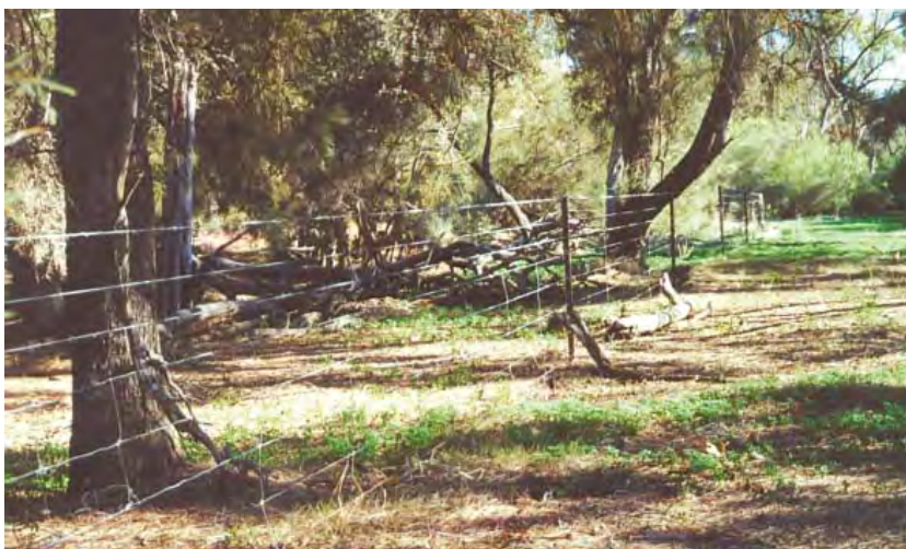
Fence condition: GOOD.
