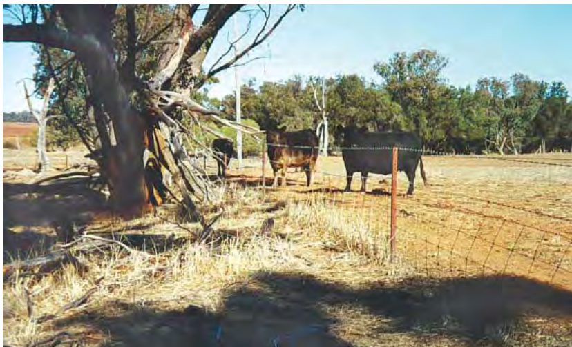
Fence condition: MODERATE.
