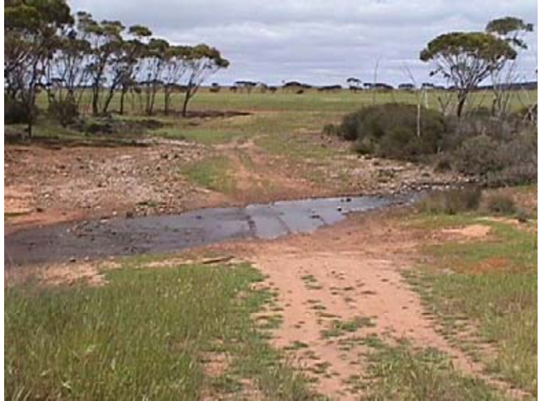
Crossing showing good design – following the contour. Small rocks could be placed to minimise the amount of water the vehicle drives through (photograph Kaylene Parker).
