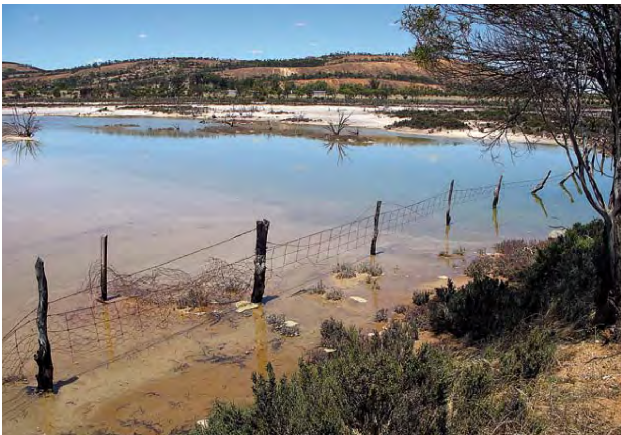
Photo 13 Water from Tropical Cyclone Clare ponding behind the Kellerberrin-Yoting Rd crossing
