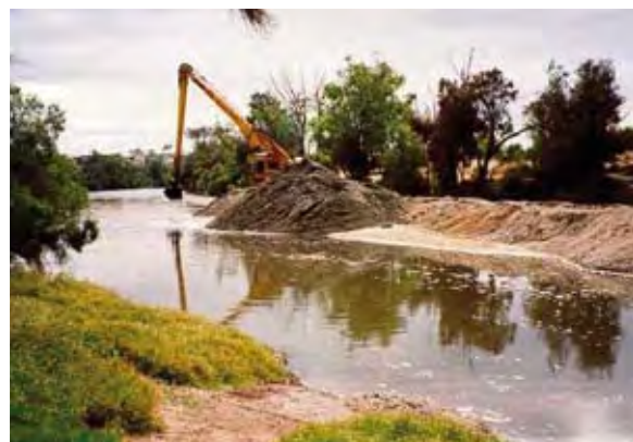
Removal of sediment from Gwambygine Pool, 1999 (Photo courtesy Peter Kata)
