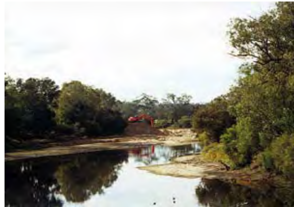
Sediment removal from Katrine Pool looking upstream (Photo courtesy Martin Revell)
