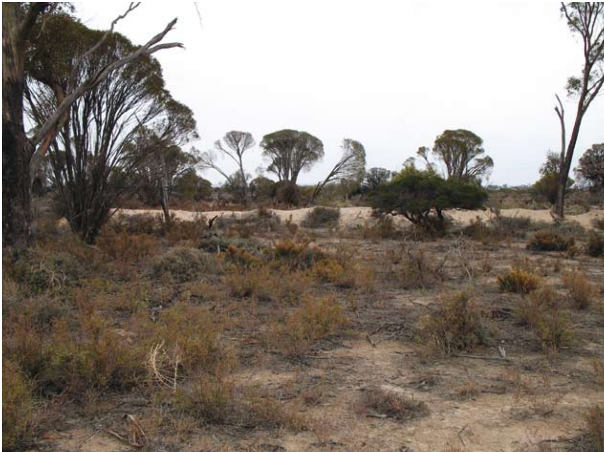
Bank constructed through Melaleuca shrubland to alleviate waterlogging problems (Photo: S. Mehmet)
