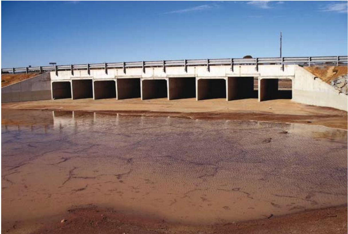
Photo 6 Culverts under Great Eastern Hwy at Baandee Lakes (Photo: S. Mehmet)
