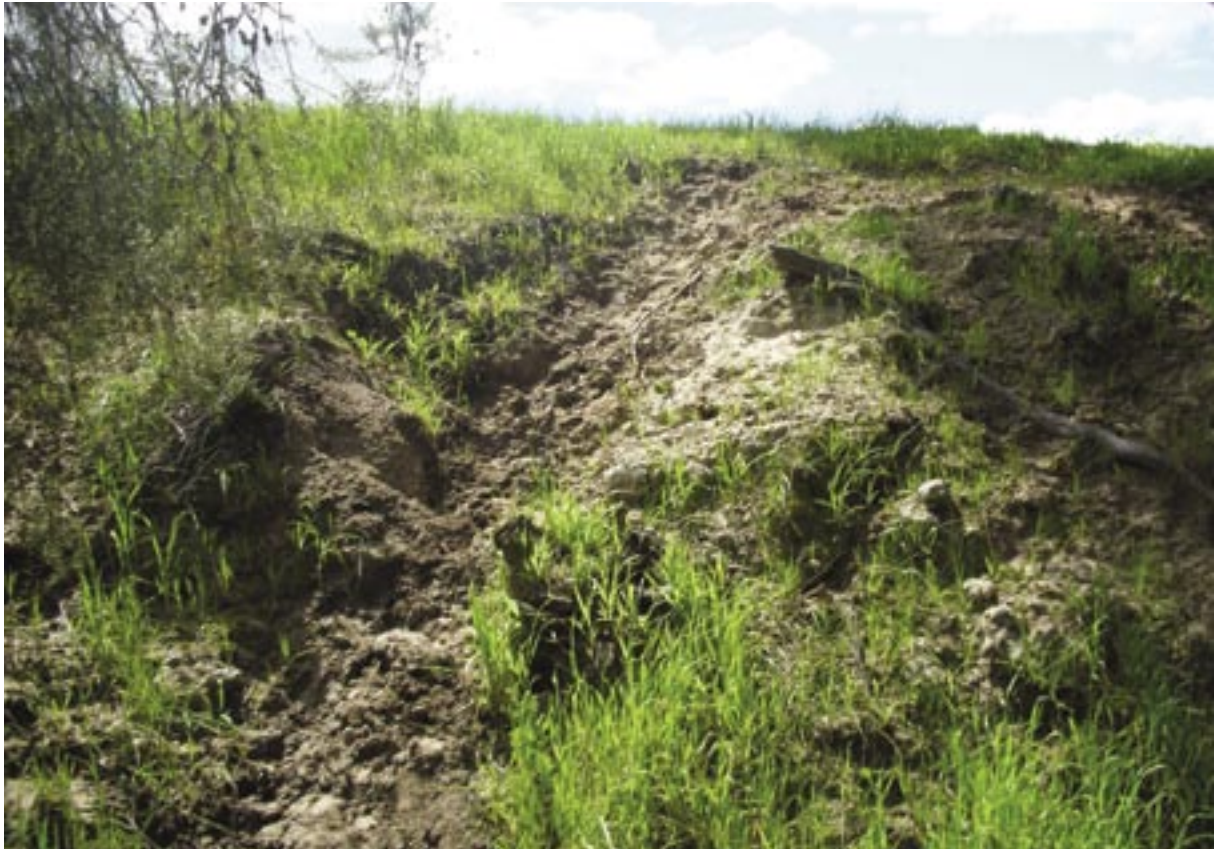
Photo 11 Stock access down this steep embankment is exposing the soil to erosion. Left unmanaged, this bank will eventually erode into the channel.
