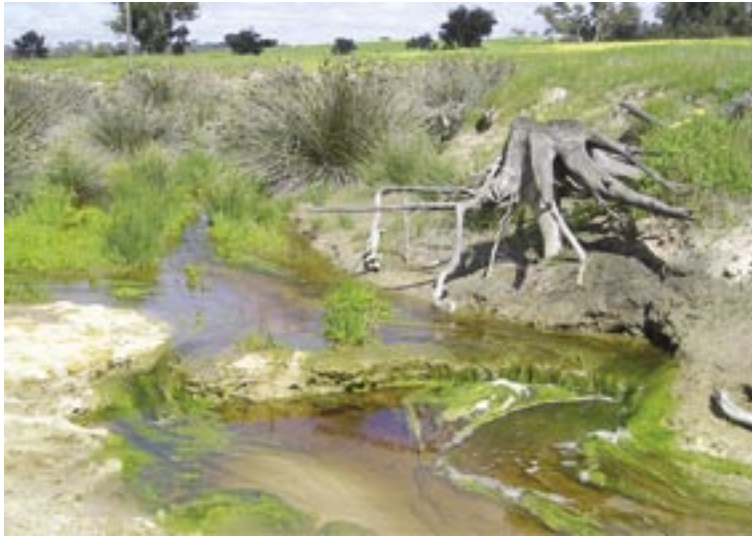
Photo 2 An exposed dead tree root along an unfenced tributary of Christopher Brook.
