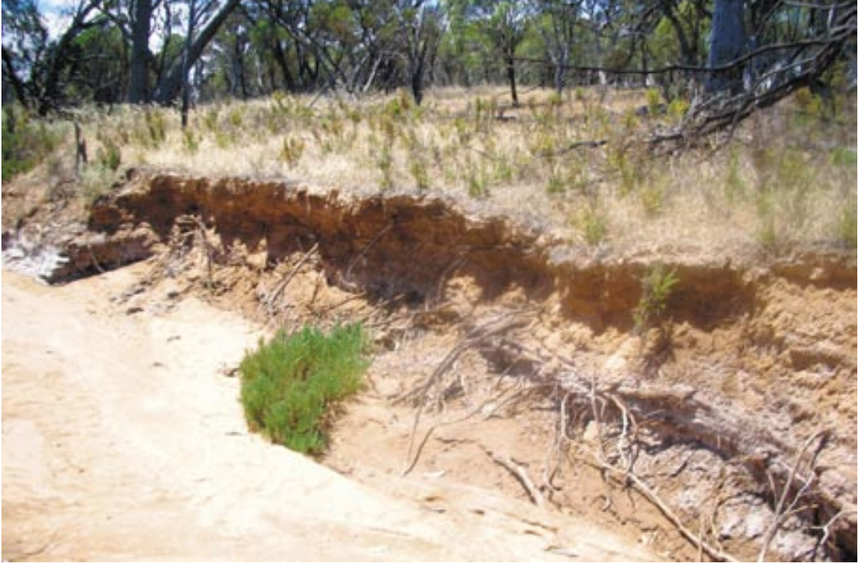
Photo 1 Bank undercutting on Monjerducking Gully
