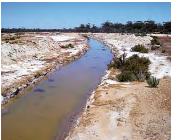
Plate A1.91: YR11 drain on eastern side of site
