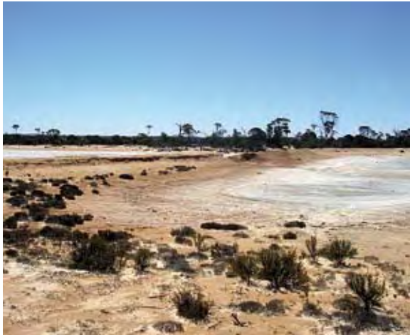
Plate A1.53: YR08 broken dam on main lake
