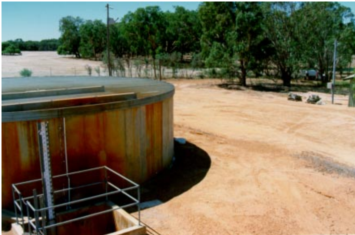
Plate 2. Water pumped from the Dandaragan wellfield is chemically treated and stored in the tank.
