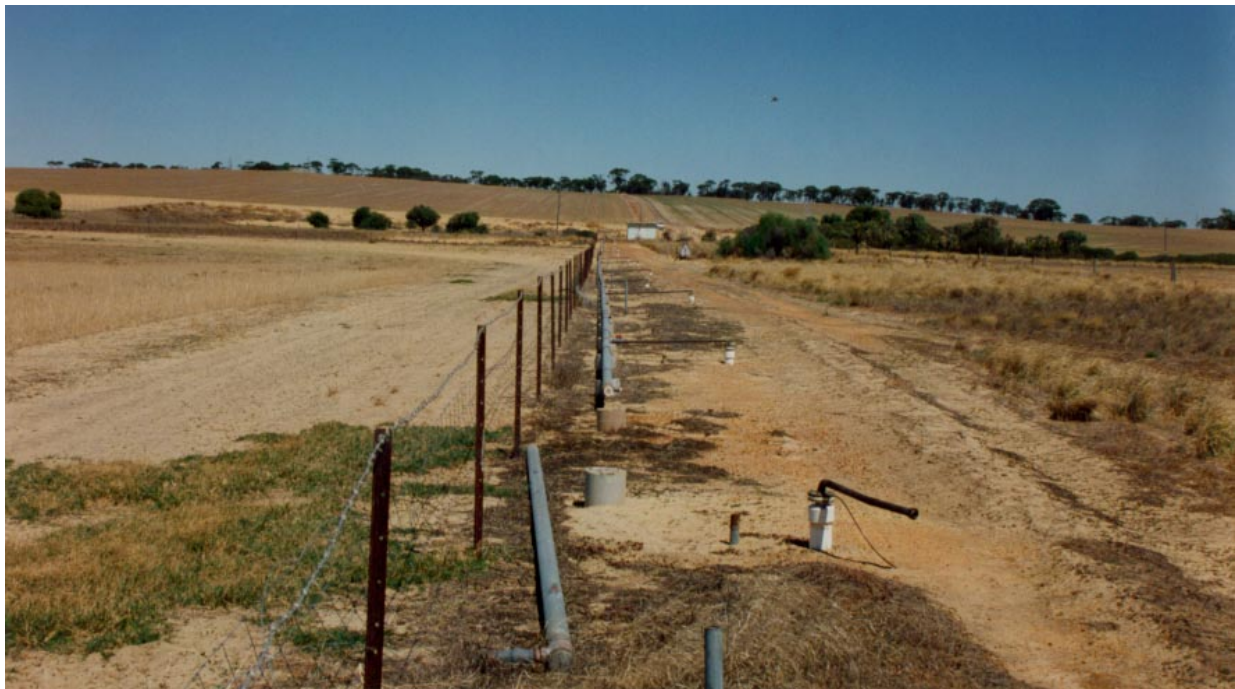
Plate 1. Yerecoin wellfield consists of a series of shallow spears 7 km east of the townsite.
