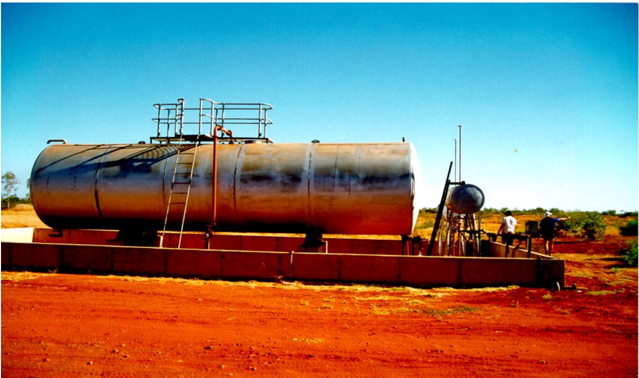
Plate 2. Bulk diesel storage at the pumping station
