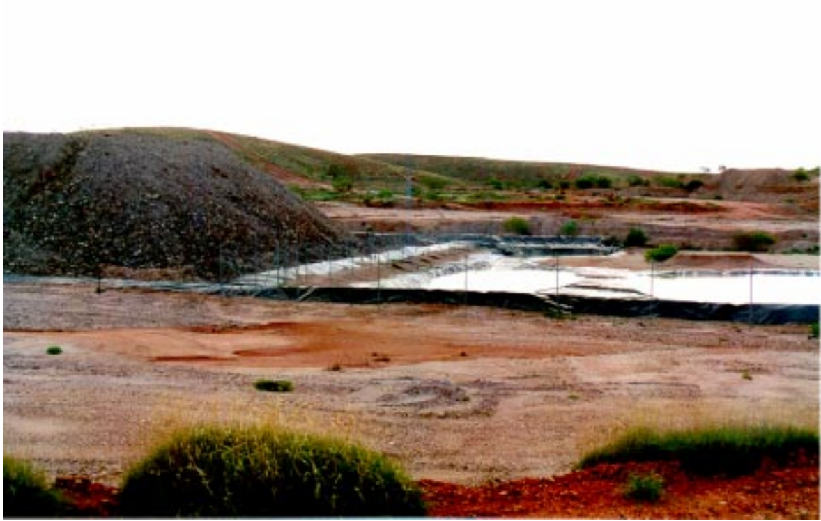
Plate 5. Cyanide leach pad at Beaton Creek
