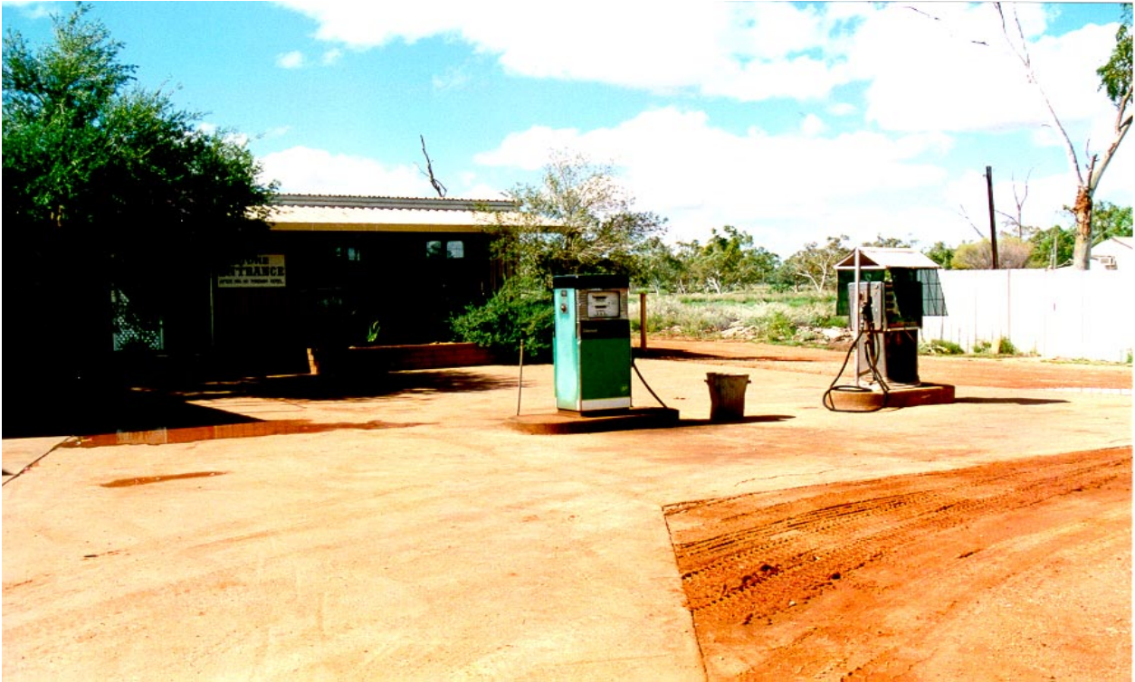
Plate 1. Underground fuel storage at the Conglomerate Hotel
