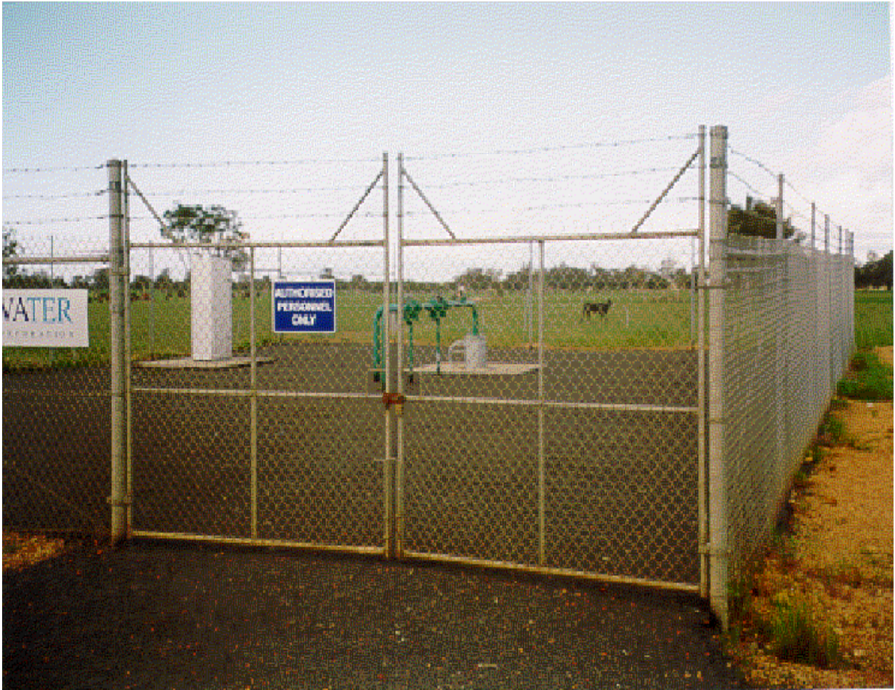
Plate 4. Typical mounting of production bores within the Quindalup wellfield
