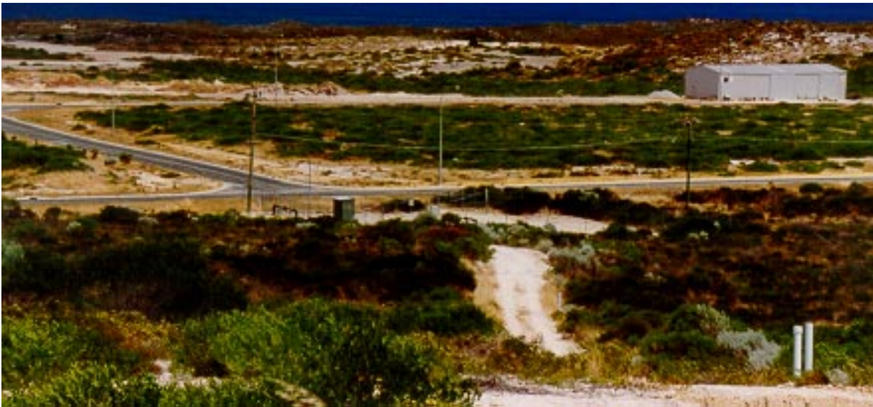
Plate 1. Light industrial subdivision at Ledge Point with wellfield on near side of road
