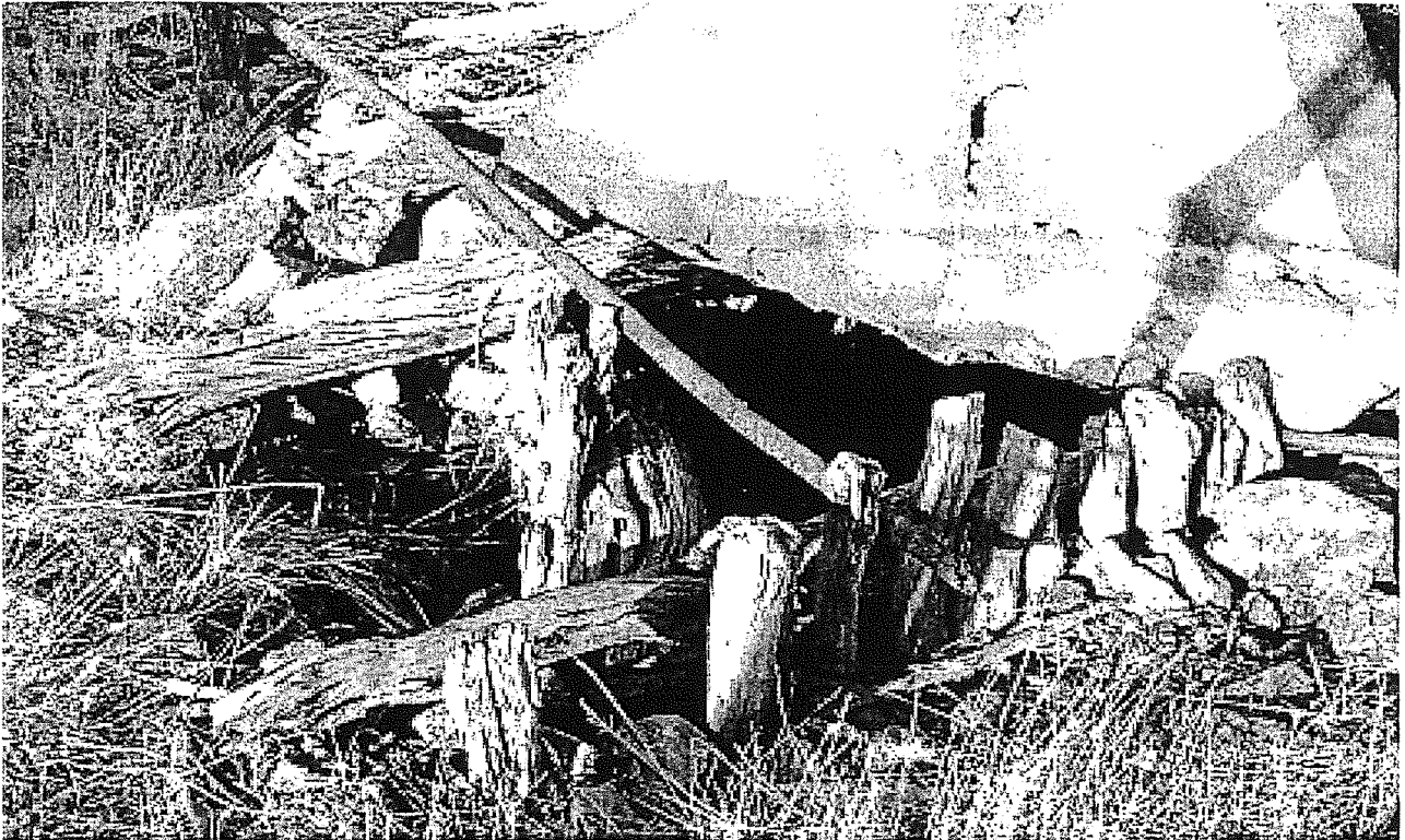
Plate 2: A poorly protected abandoned well adjacent to a production bore
