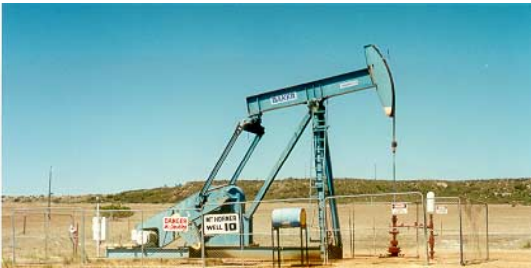
Plate 2: Oil production well, Mt Horner oilfield.
