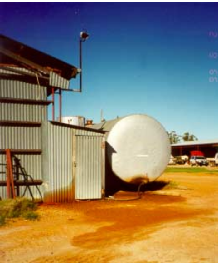
Plate 4: Evidence of fuel spillage (tank and contaminated soil now removed), Allanooka Farm, Mt Horner West Road.
