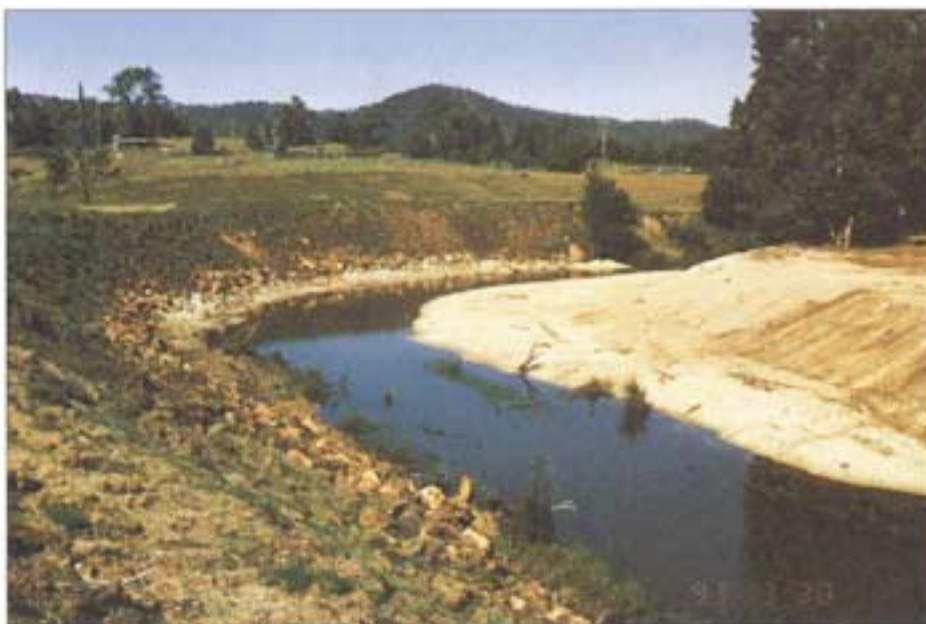
Plate 39. View of a riverbank revegetation trial. The gravel bench between the low-flow channel and a rock revetment has been densely planted with seedlings of Waterhousea floribunda .
