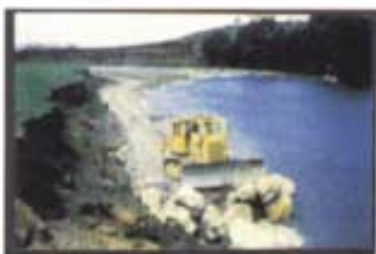
Rock toe protection
