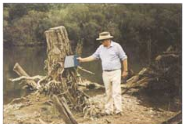
Plate 38. Example of a site where vegetation has been trimmed at a break-out point and the decrease in hydraulic roughness resulted in removal of bed material, thereby increasing the main channel capacity. The folder marks the original bed level. The remaining roots control the process.
