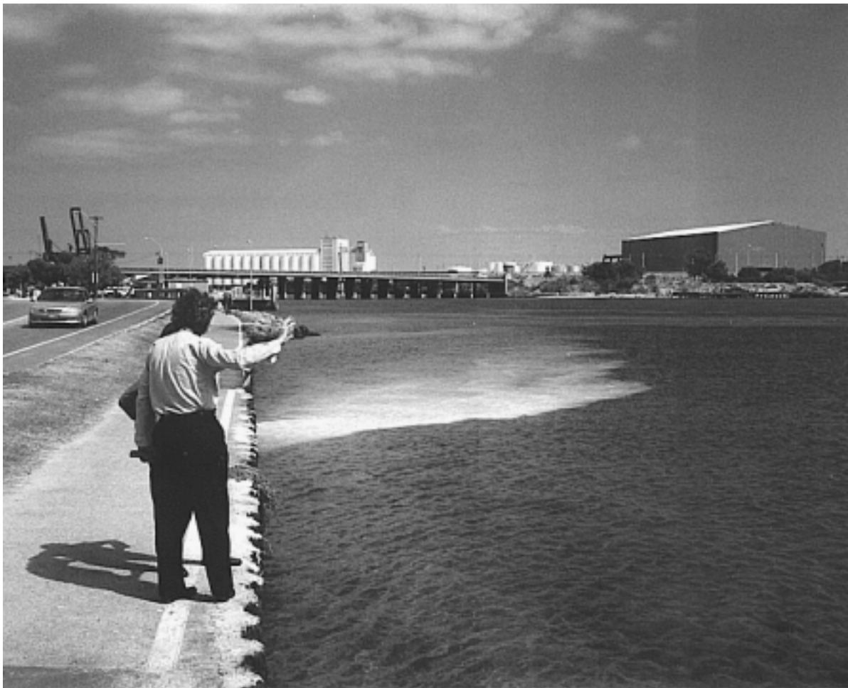
Sediment plume from dewatering operation, East Fremantle.
