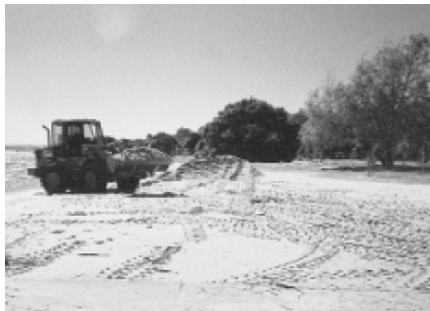
SRT crew 'renourishing' eroded beaches with sand from beaches with a surplus supply.
