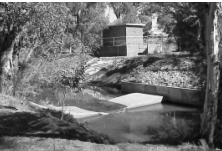
A high quality gauging station at Canning River, Seaforth Avenue (accuracy of flow data +/- 5%).
