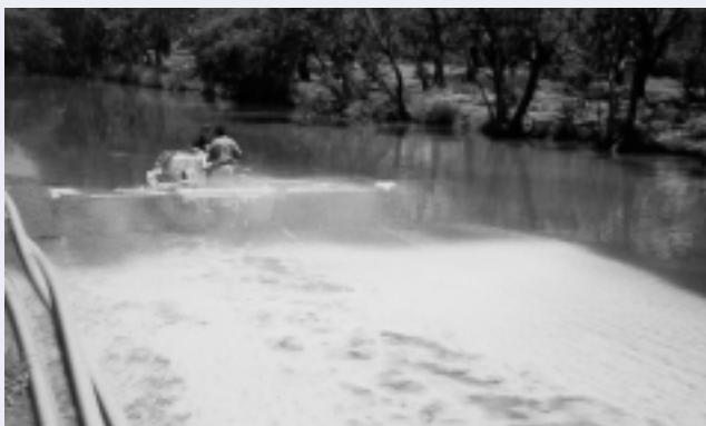
PhosLock™ being applied as a slurry to the Canning River.
