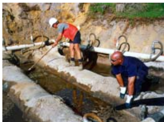
Liquid waste tanker removing diesel fuel from a hole located opposite Cloisters Boat Ramp in Manning.
