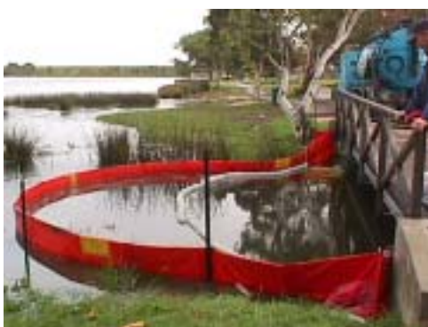
Trust field crew used absorbent spill booms to contain a diesel spill before it entered the Swan River in Belmont on 2 July 2000.
