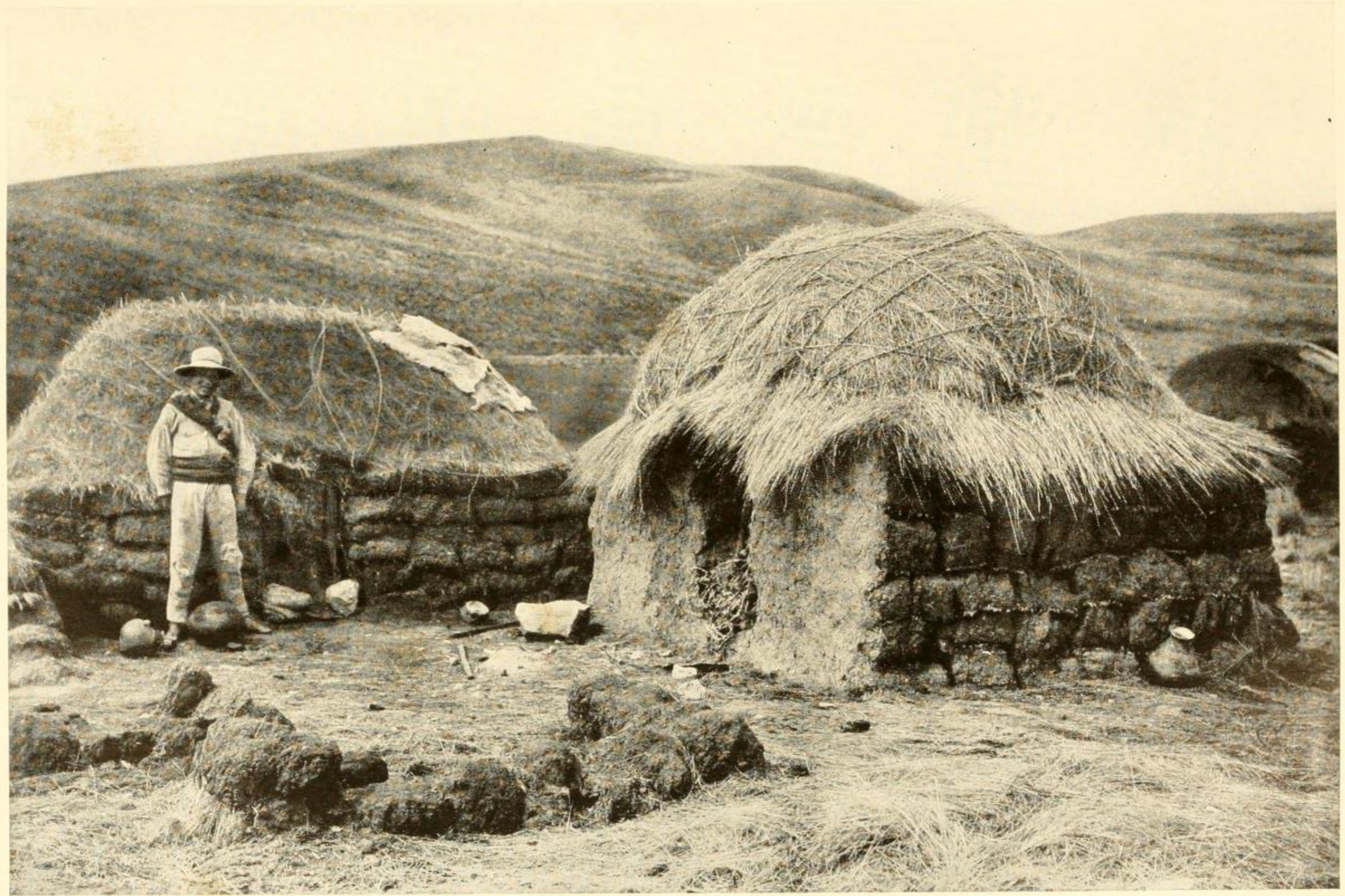
Sheep herders' huts in the high Andes, Peru (13,000 feet). The walls are of sod. The roof, of ichu grass ( Stipa ichu ), is held down by ropes. Photograph by Hitchcock
