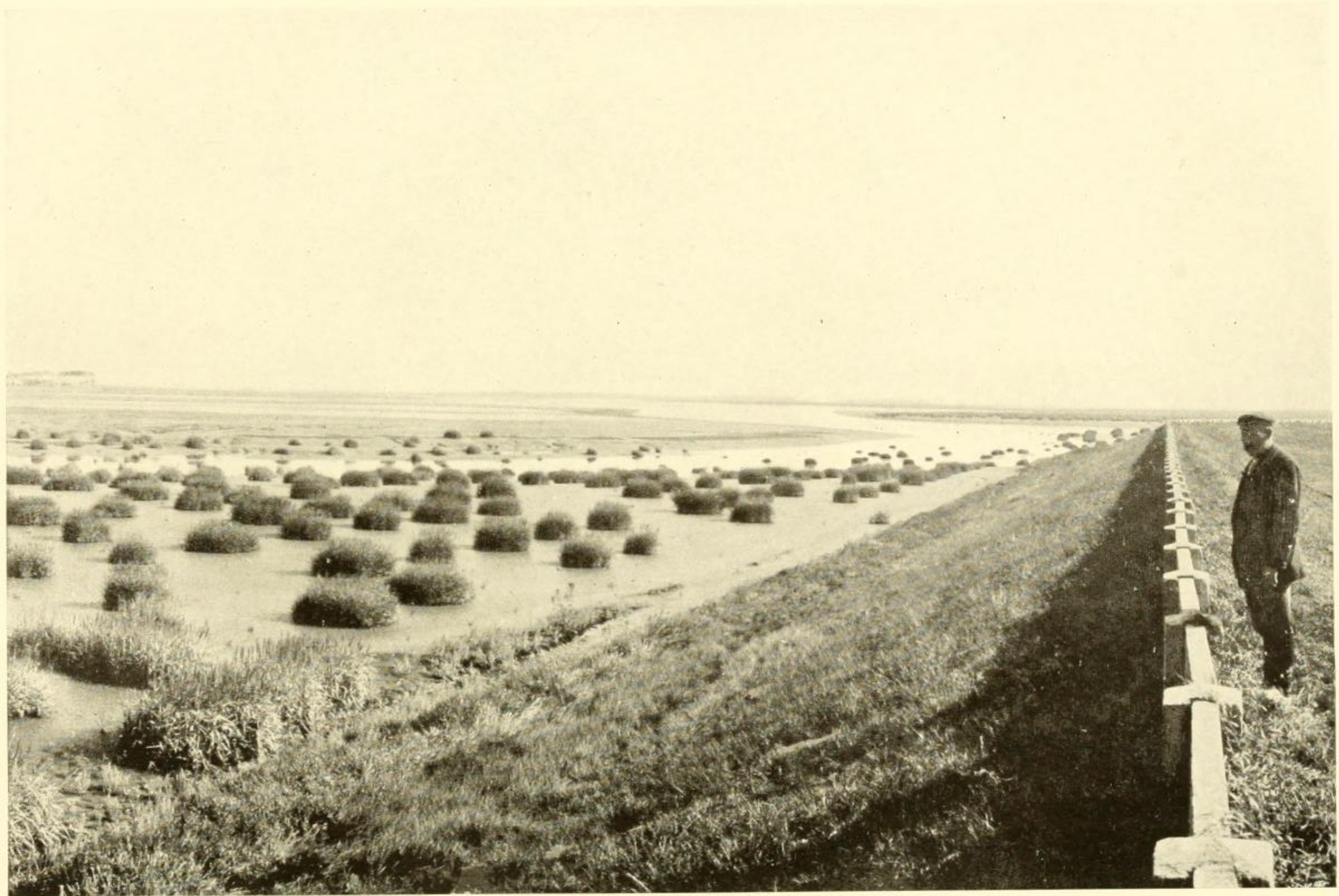
Spartina Townsendii building land outside a dike in the Netherlands. Photograph by Prof. F. W. Oliver, of London
