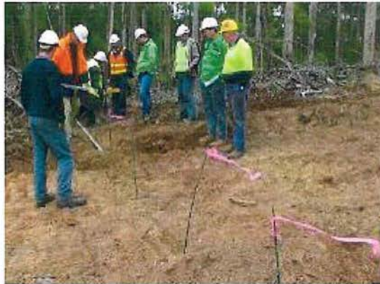
1. Pegging the alignment
