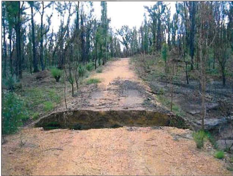
Figure 9: After a fire, the combination of increased overland flow of water together with reduced soil stability and ineffective road drainage structures can result in severe erosion events.
