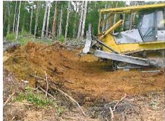
2. Cutting and pushing the bank
