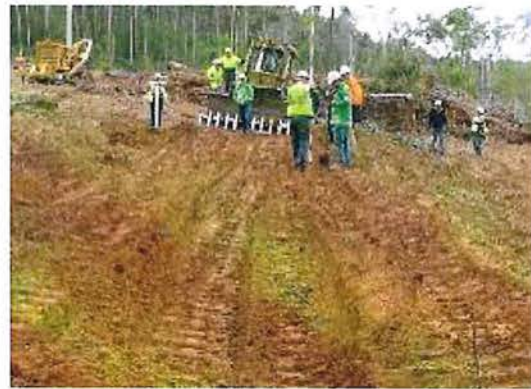
4. Inlet and outlet cleared and compacted
