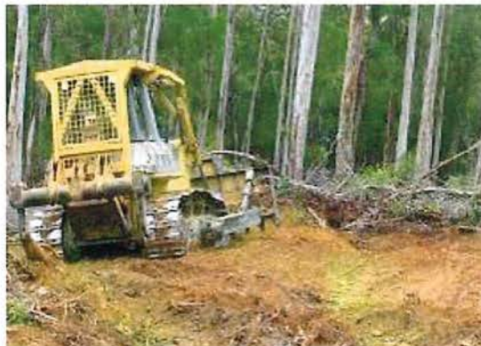
3. Compacting spoil on the bank
