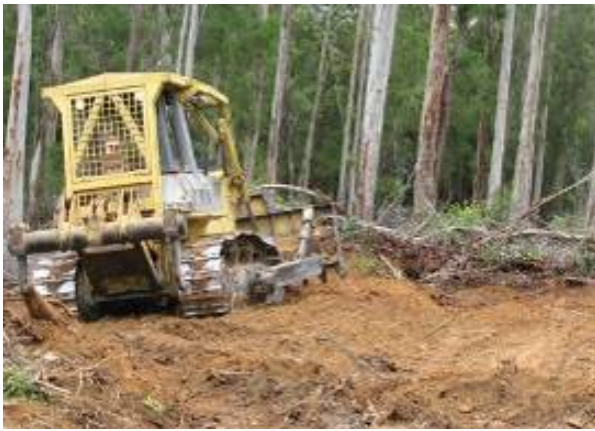
3. Compacting spoil on the bank.
