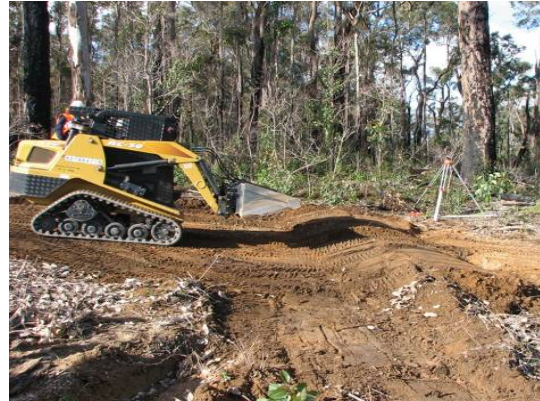
Rolling dip construction using a bobcat
