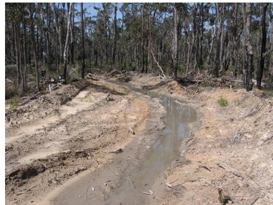
Outlet from a relief culvert on Crouch Road
