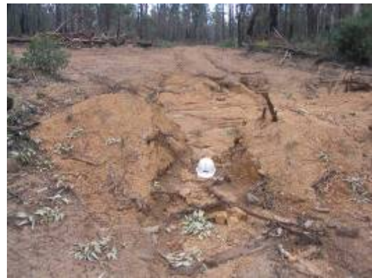
Figure 7: Damming can result in catastrophic failure due to overflowing
