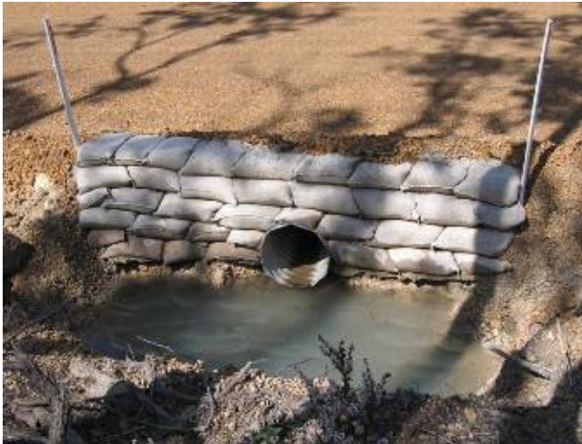
Figure 17: A culvert inlet and inlet sump.
