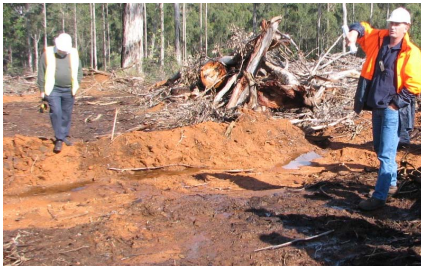
Figure 8: An example of a spreader that is well constructed with an outlet that moves water off the extraction track to a stable surface.
