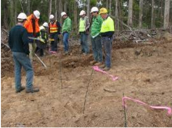
1. Pegging the alignment.
