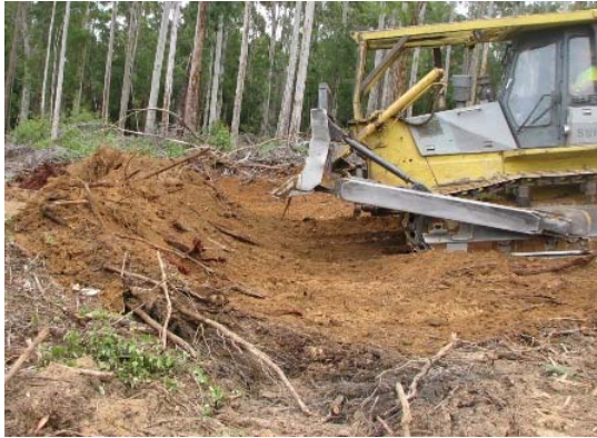
Rolling dip construction using bulldozer
