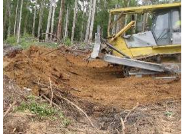
2. Cutting and pushing the bank.
