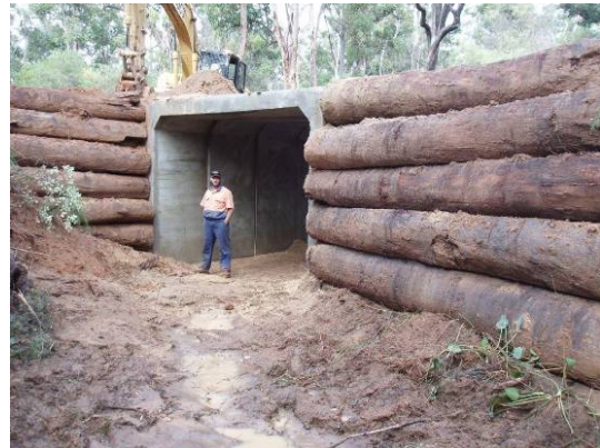
Box culvert replacing a previous bridge on Crouch Road.
