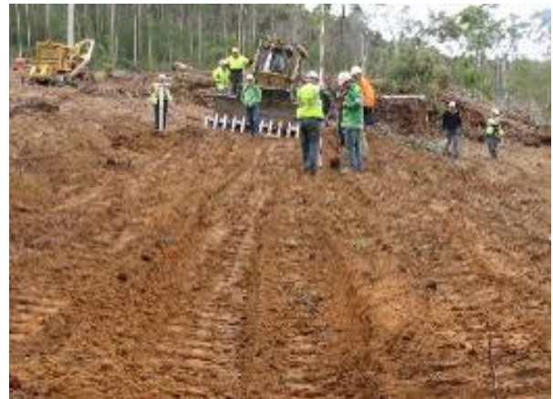
4. Clearing and compacting the inlet and outlet
