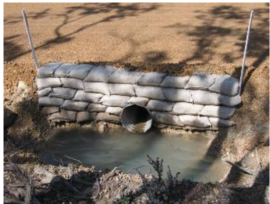
Inlet end of relief culvert on Crouch Road.
