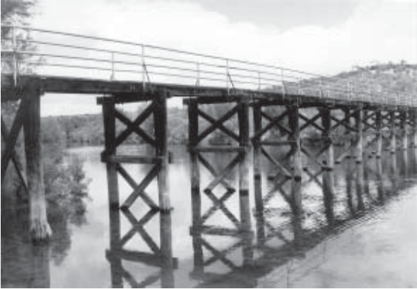
Poole Street Bridge. [Photograph courtesy of C Ryan]
