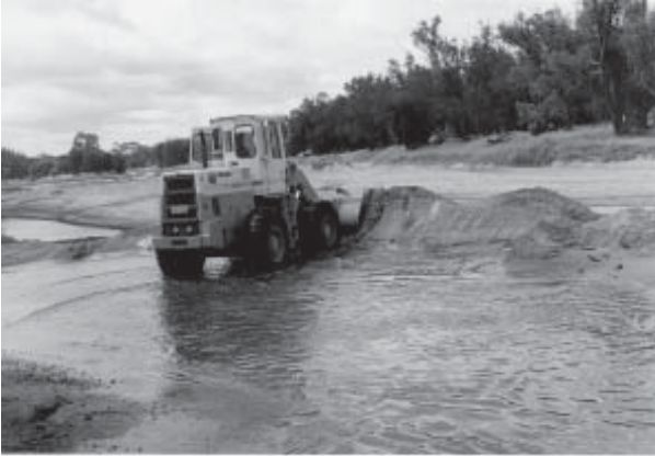
Excavating sediment traps, Burlong Pool. [Photograph courtesy of C Ryan]
