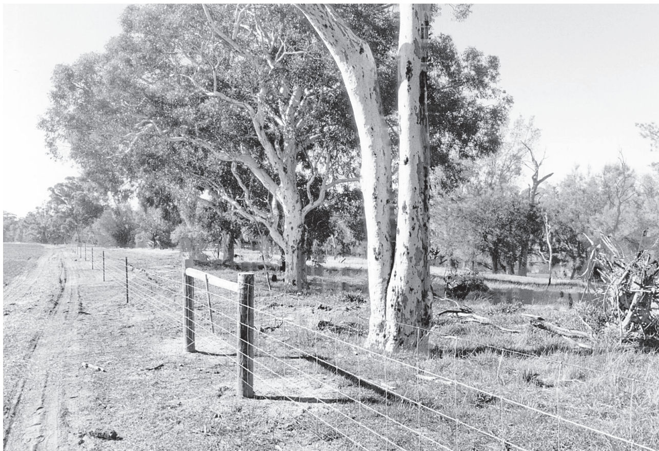
Fencing along the Avon River
