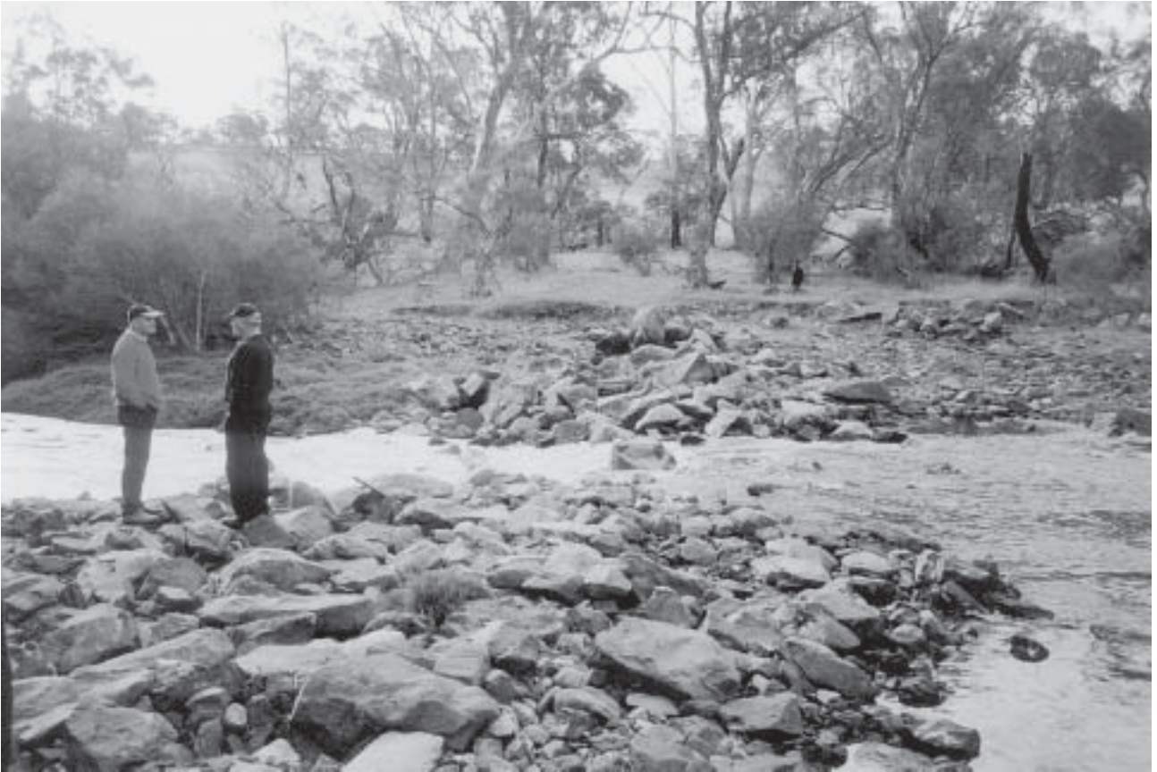
Photo 7: The river bed elevation difference maintained by Glen Avon Weir
