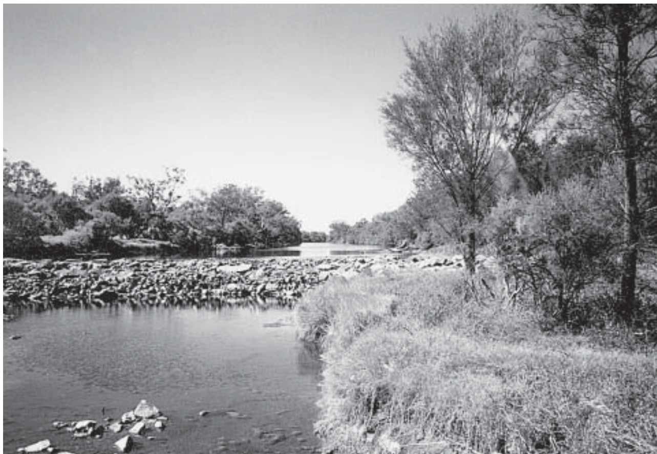
Photo 6: Glen Avon Weir
