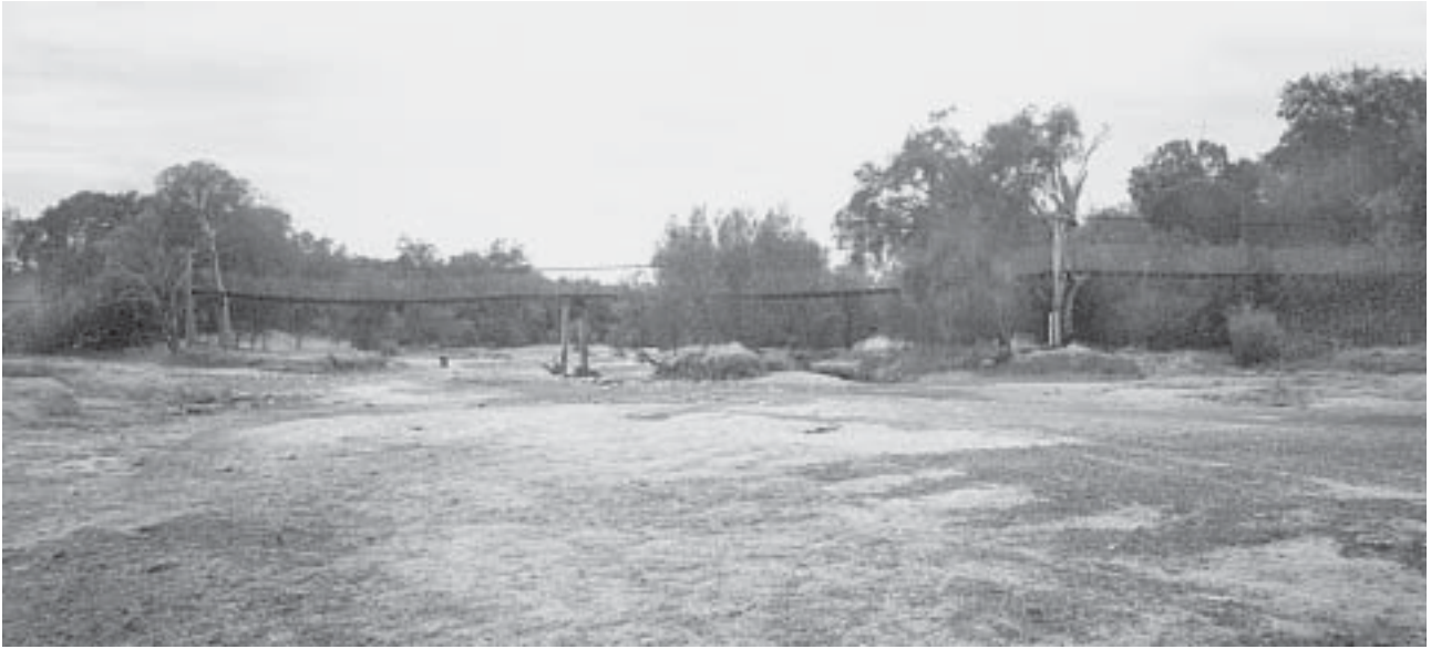
Photo 17: The Swinging Bridge at Muresk
