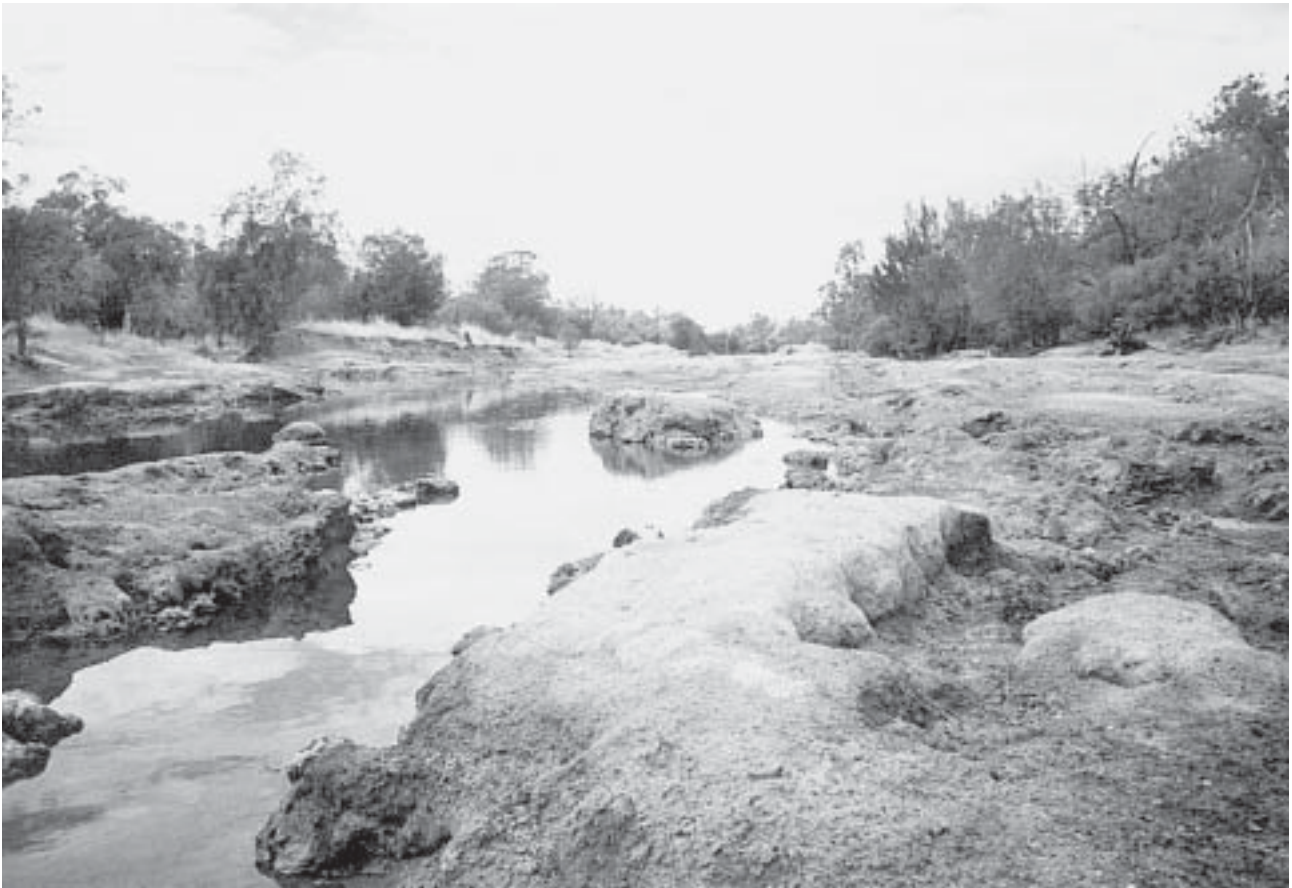
Photo 3: The scoured river channel after the training scheme
