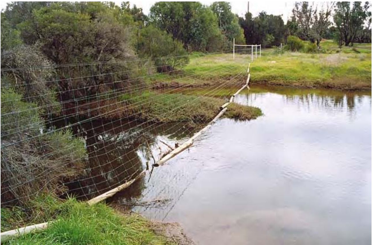
Image 9. A well-constructed, well-maintained cross-channel fence
