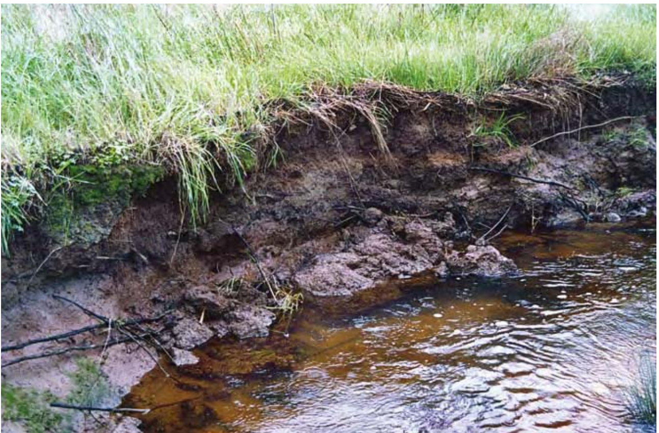
Image 3. Slumping, where an undercut bank has collapsed under its own weight
