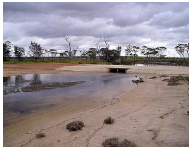
Photo 32: Substantial farm access crossing in Photo Section 18
