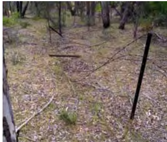
Photo 27 Fencing in poor condition adjacent to the rail corridor
