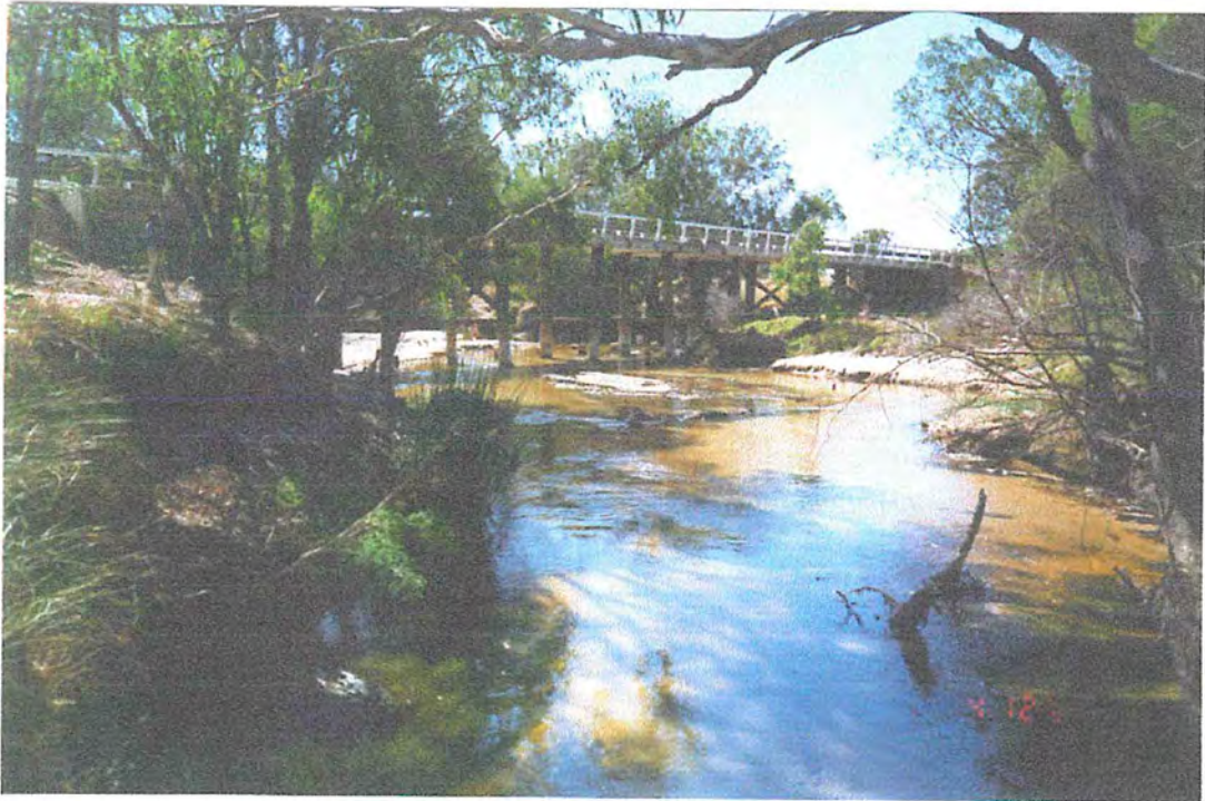
Photo 12 Moore River flowing beneath Cowalla Bridge, 07/02/01
