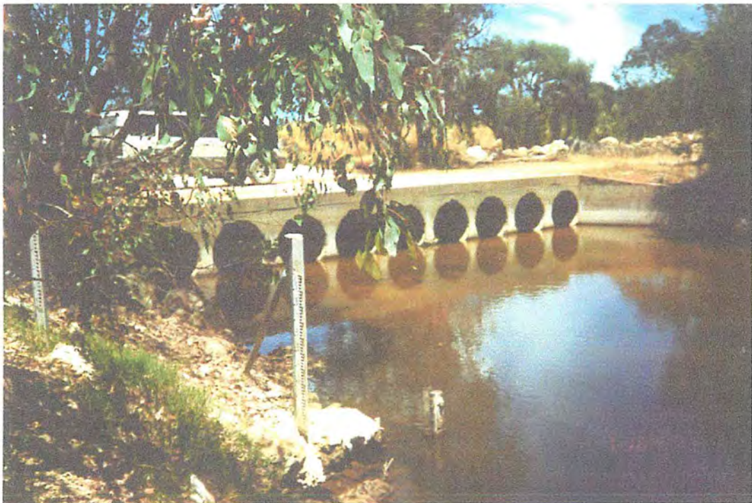
Photo 8. Bennies Road. Flood gauging station on east bank. High salinity area. Paper barks ( Melaleucas ), which favour a high groundwater table, growing on the east side of the river, 15/11/00.
