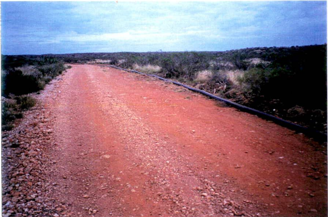
B. A typical newly-constructed access road. The width is required for equipment access during construction. Once installed the vegetation grows back on the sides until the track is only a car width. The polypipe has been laid on the surface and is identical to that proposed for the extensions.
