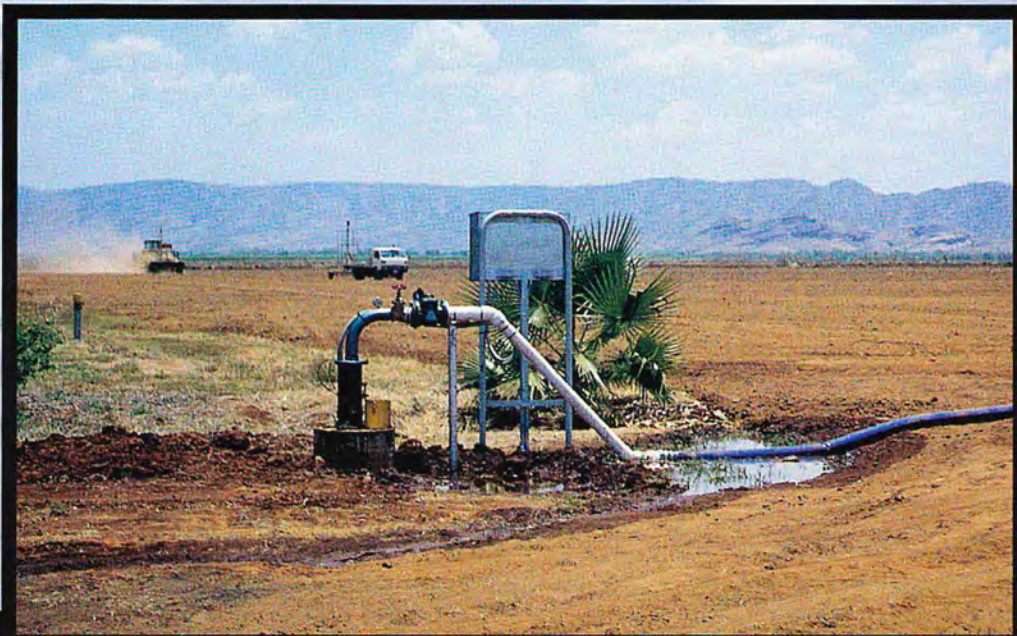
Photo 1: Ground water trial pump bore at Bardena Farms
