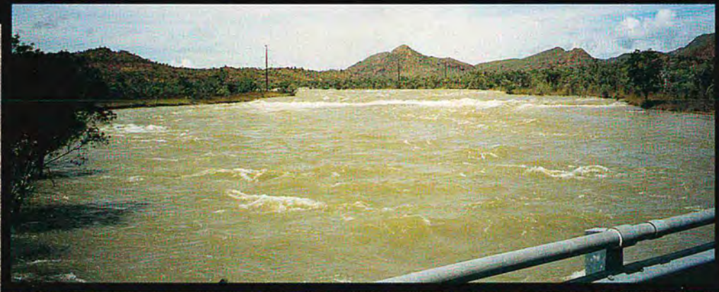
Photo 9: Flow down the Lake Argyle spillway – March 2000
