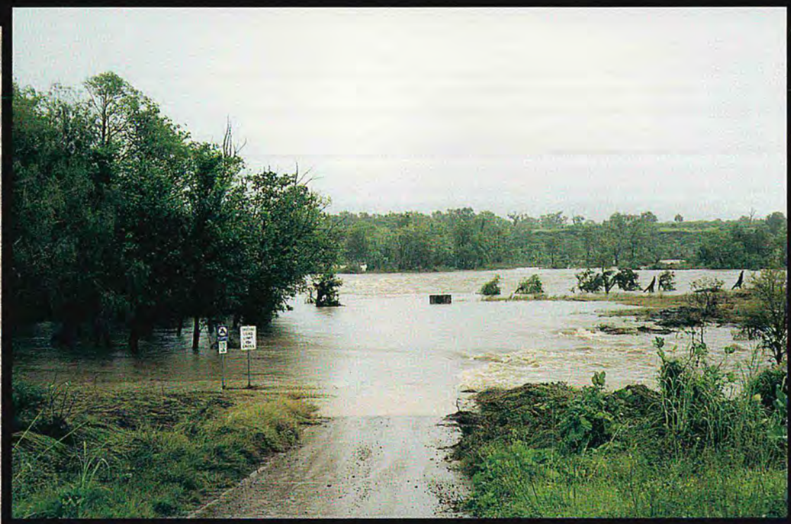
Photo 7: Ivanhoe Crossing with the Ord River in flood on March 5th 2000
