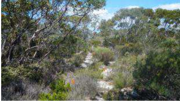
Pre-construction – approaching machine slasher just visible in distance (5 October 2012)
