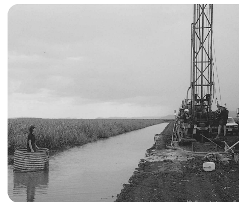
Drilling monitoring bores, Ord River Irrigation Area
