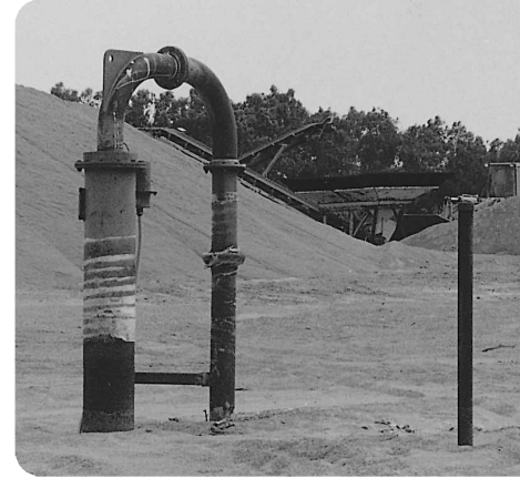
Submersible pump near mining sand tailings, Gascoyne
