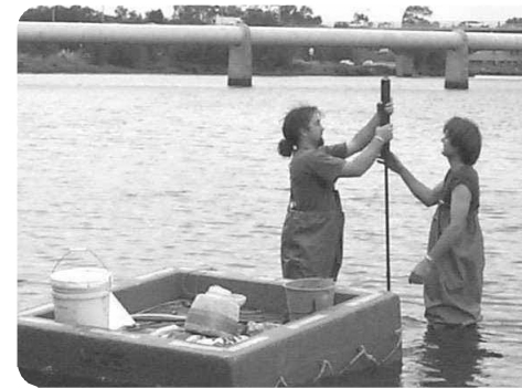
Installing groundwater monitoring bores in the Canning River
