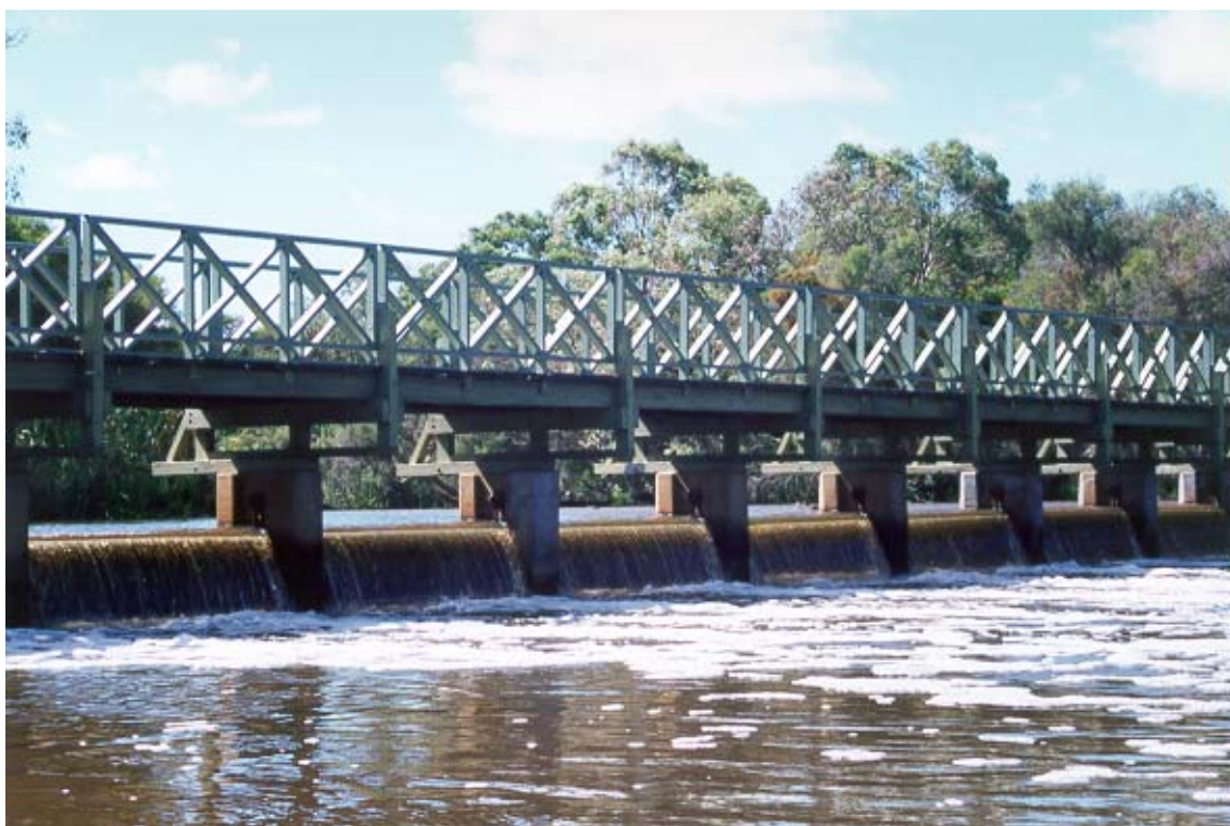
Kent Street Weir, Cannington
