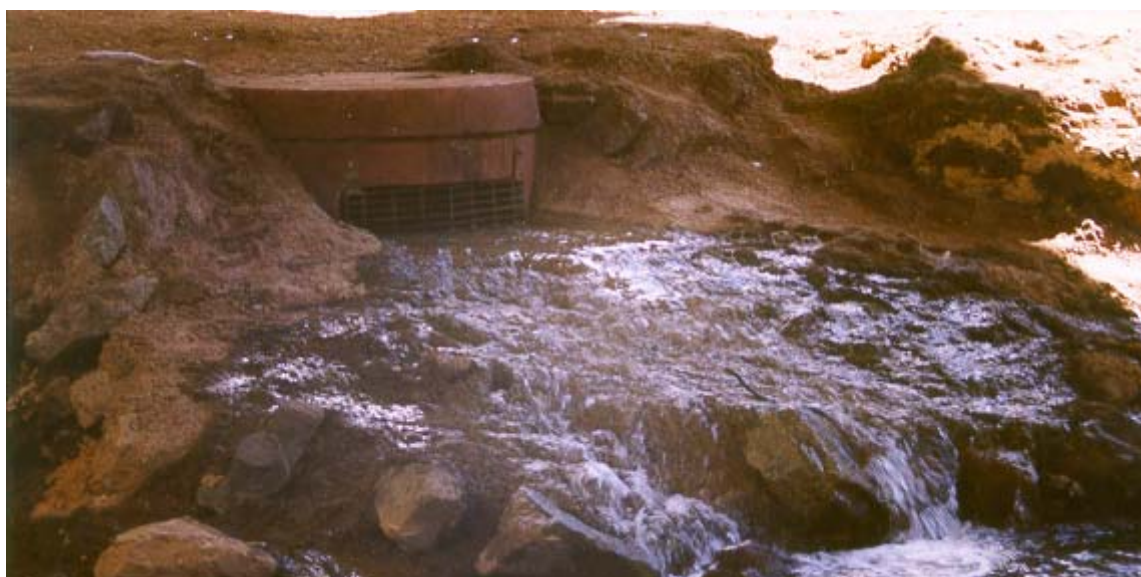
Environmental release point, Albany Highway Bridge, Gosnells
