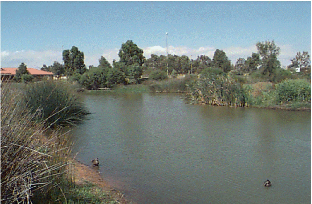
Stormwater detention basin
