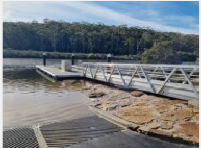
New jetties on the Frankland River
