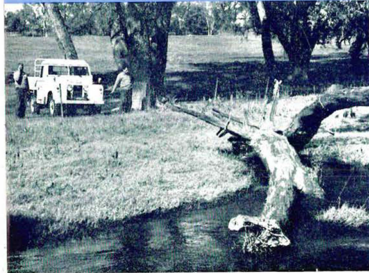
De-snagging in the Helena River. Snags are winched to the foreshore, cut up with a chain saw and burned.
