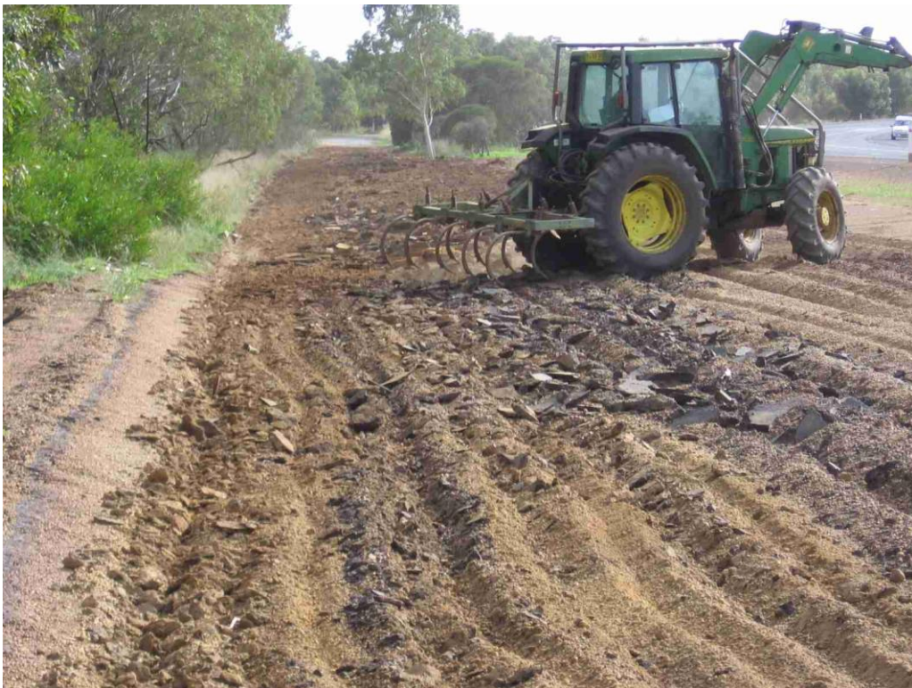
Tines preparing previously ripped road surface for seeding.
