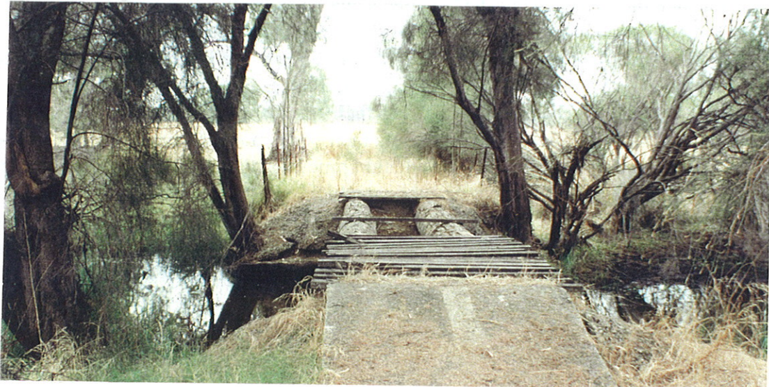
Cutaway Bridge Bennett Brook Photograph: K. Pearson
