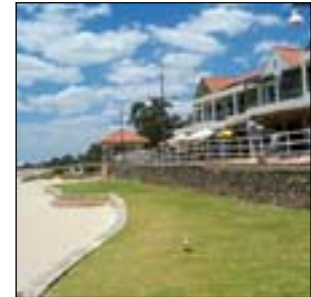
Old Rockingham town centre foreshore redevelopment
