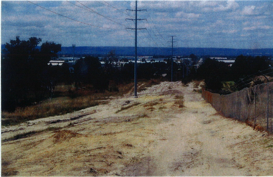
Fig 6 Recently constructed transmission line.
