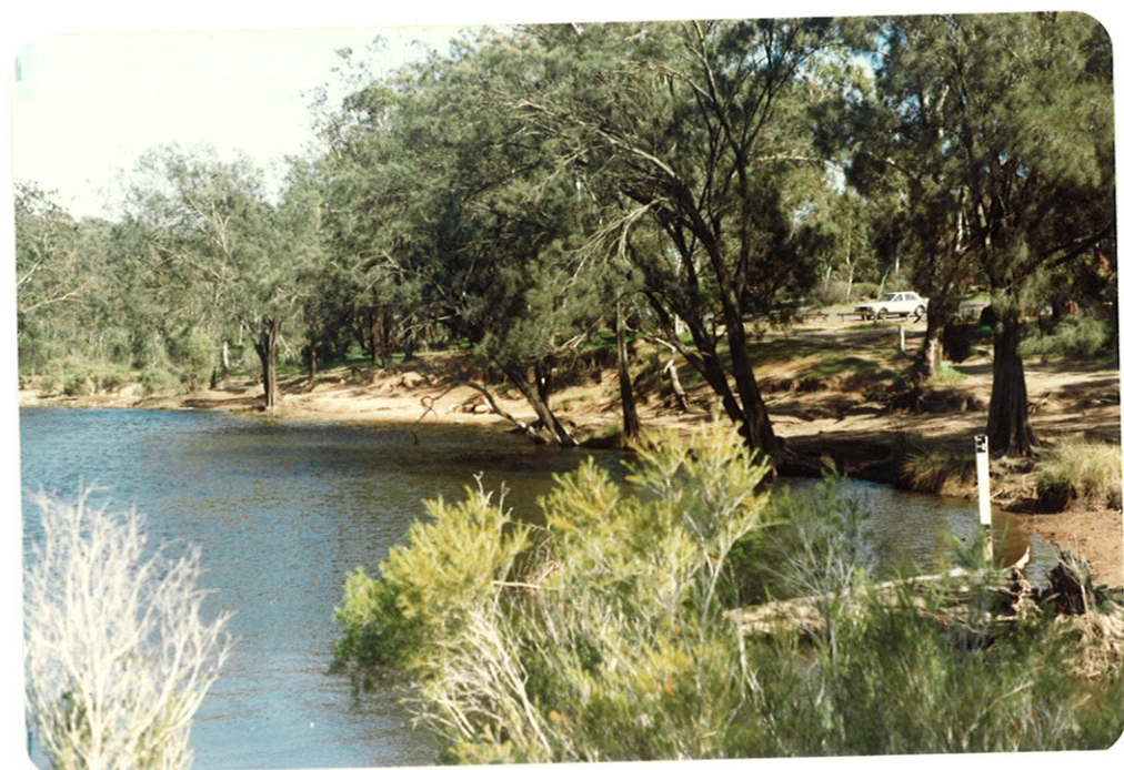
View of bank erosion down slope from carpark.
