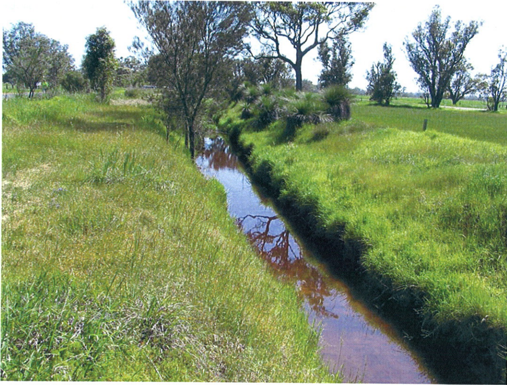
Figure 28: Dowdells Line Road drain from approximate discharge point, looking north
