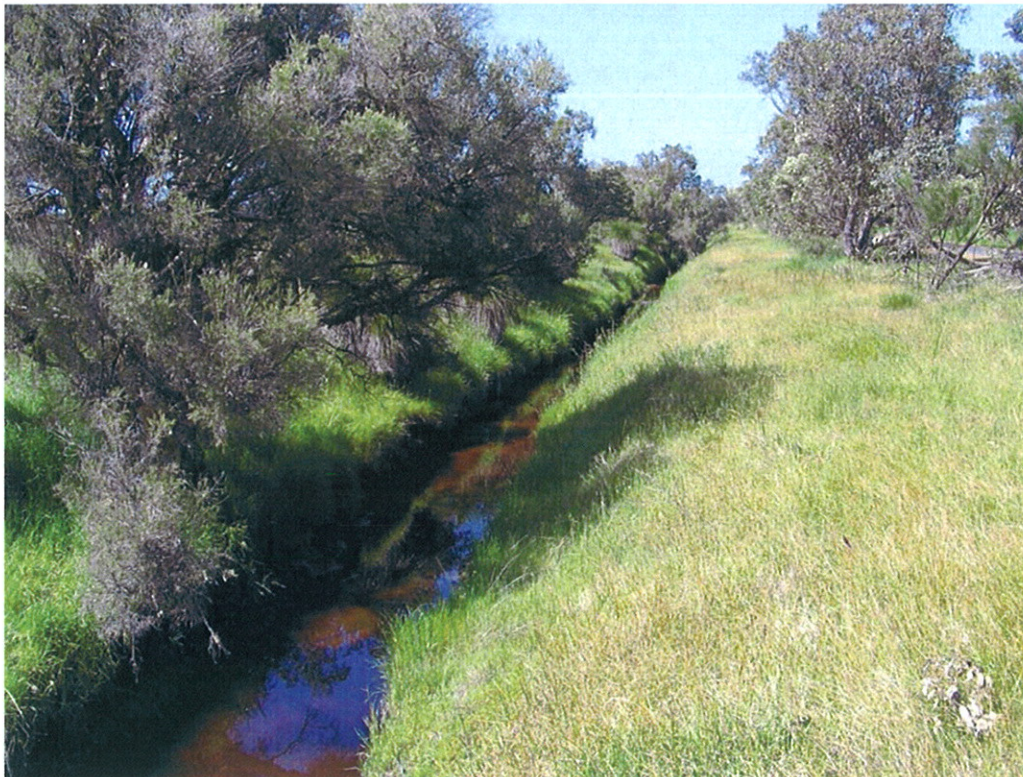
Figure 27: Dowdells Line Road drain from approximate discharge point, looking south
