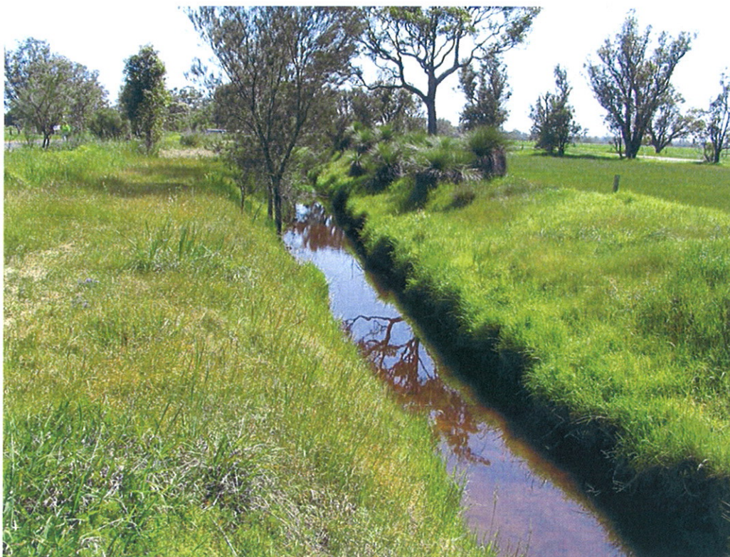
Figure 19: Dowdells Line Road drain from approximate discharge point, looking north
