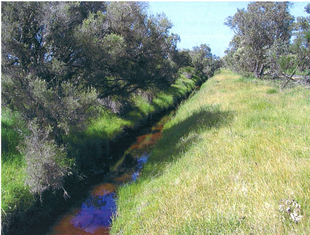
Figure 18: Dowdells Line Road drain from approximate discharge point, looking south
