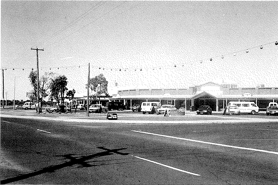
14. New Dunsborough Shopping Centre.
